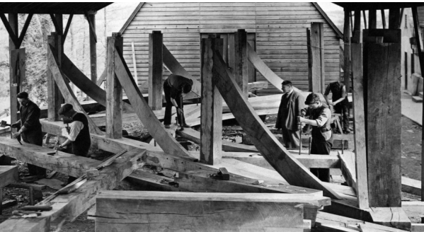
Photo: Reconstruction of the Great Hall: making the beams for the hammer beam roof. (Copyright Dennis Mill, Cirencester)
